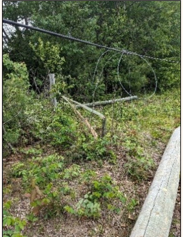
Aftermath of significant storm damage in the Petawawa training area.
