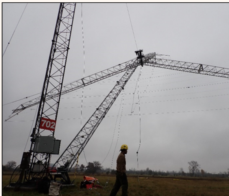
Lowering the pivot tower of a 89J to conduct maintenance.
