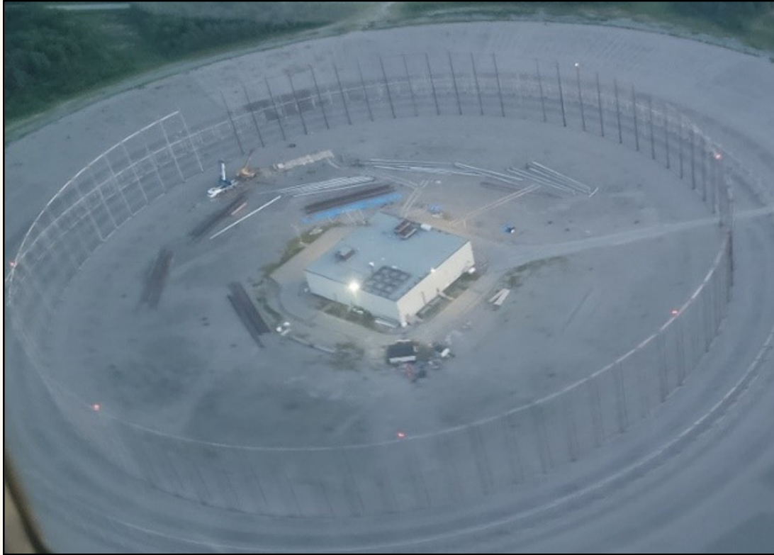
FRD -10 Antenna Structure being replaced
