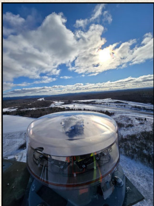
New obstruction light install, Gagetown RTA
