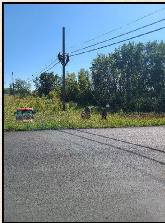
From left to right: Members of tower crew working on 100ft tower and line crews working on re-lashing bays
