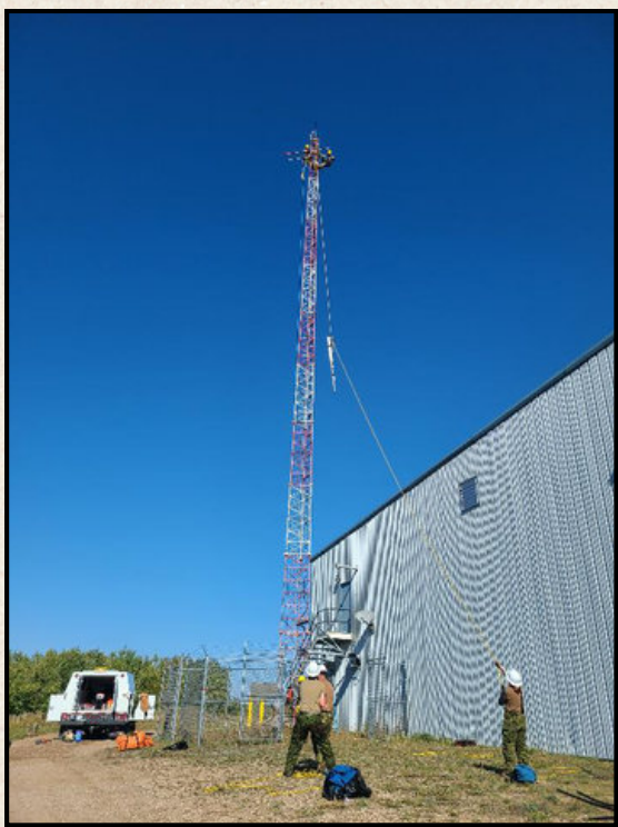
From left to right: Members of tower crew working on 100ft tower and line crews working on re-lashing bays
